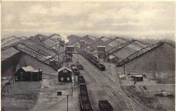
Fig. 3. Shear-Truss Construction Invented as a result of the Rondout experience; Susquehanna Coal Co.'s Plant at Old Bridge, N. J.
